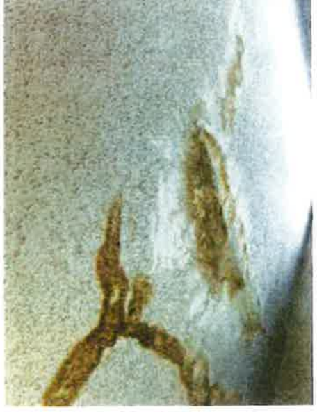
Photo 4: Knights Inn Ceiling Surface Material (HA-04)
