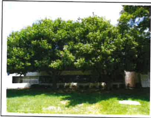
Building Exterior South
