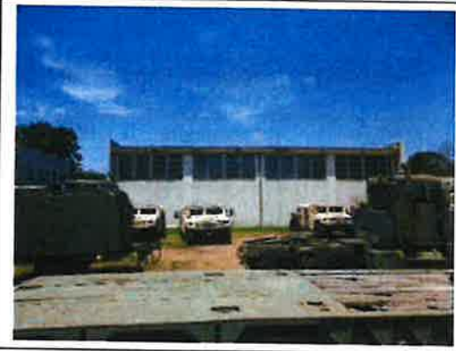
Building Exterior East
