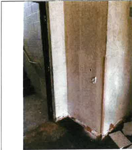
Sample 01 – Sheetrock/joint compound foyer downstairs
