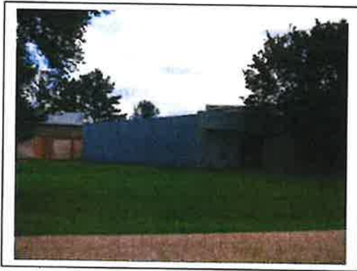
Building Exterior West
