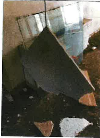
Sample 04 – 2x4 ceiling tile
