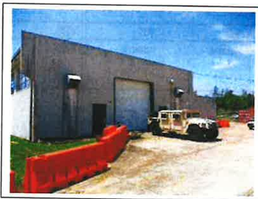
Building Exterior North
