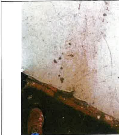
Sample 05 – staircase epoxy/paint
