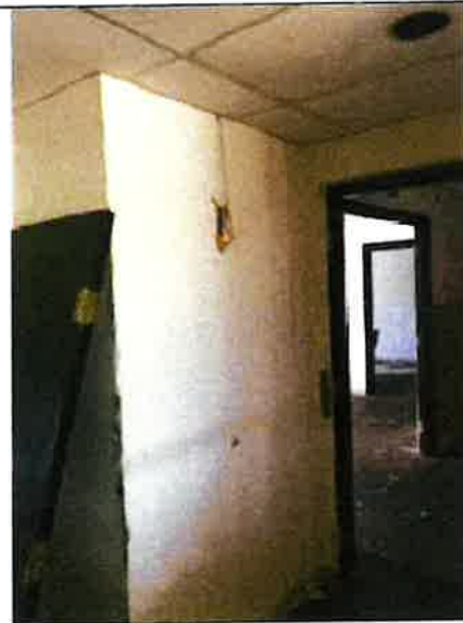
Sample 02 – sheetrock front office
