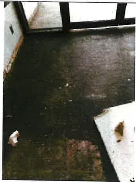
Sample 03 – Black mastic-front foyer
