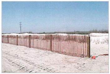
Figure 1 Sand Fence (http://www.gulfmex.org/crp/7004/fence.jpg)
