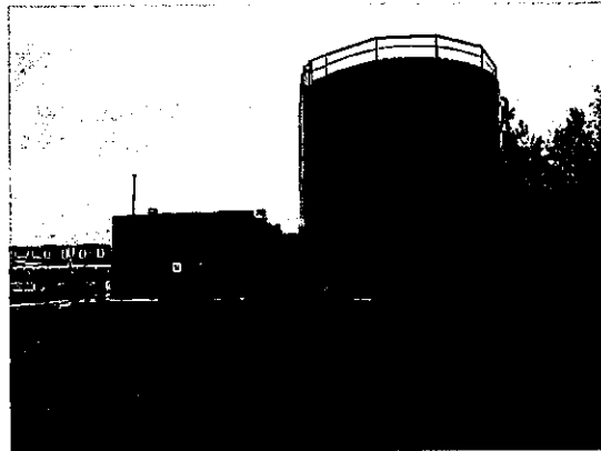
Emergency Water Tank
