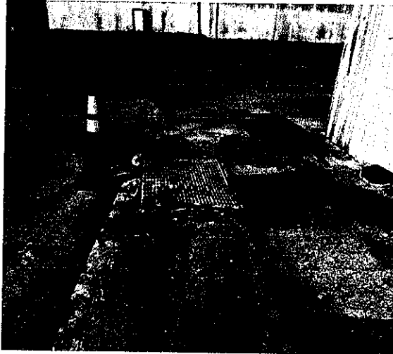
Photo 7: Stormwater trench and drain
