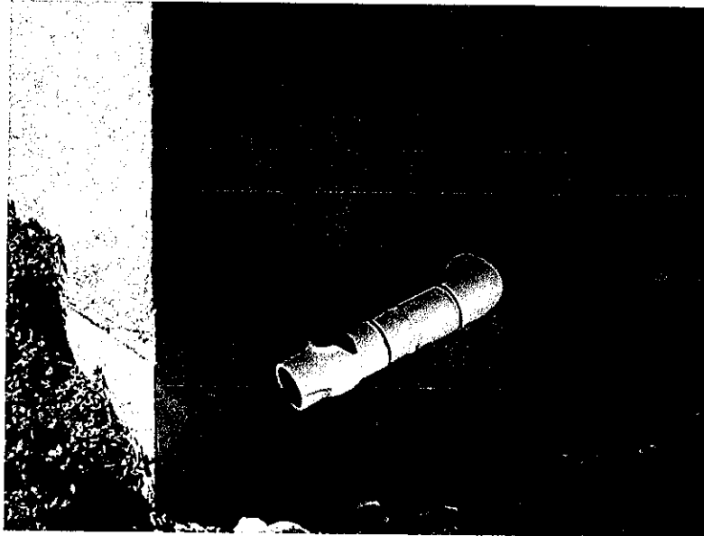
Photo 4: Stormwater Drain from Secondary Containment
