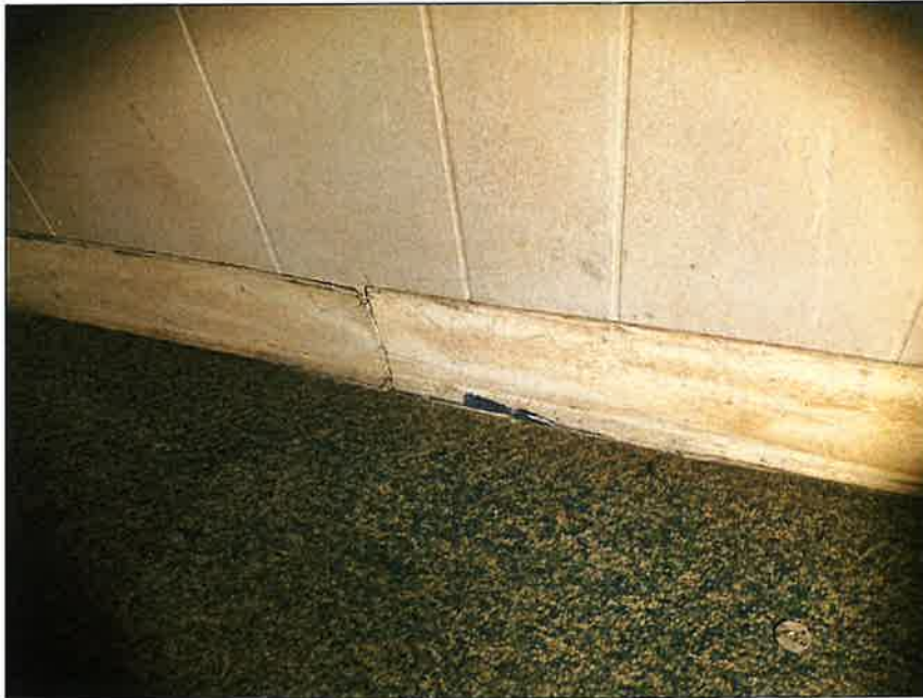
36 - Eastern Structure - Non-ACM 4" White/Blue Cove Base and Mastic (CB1)
