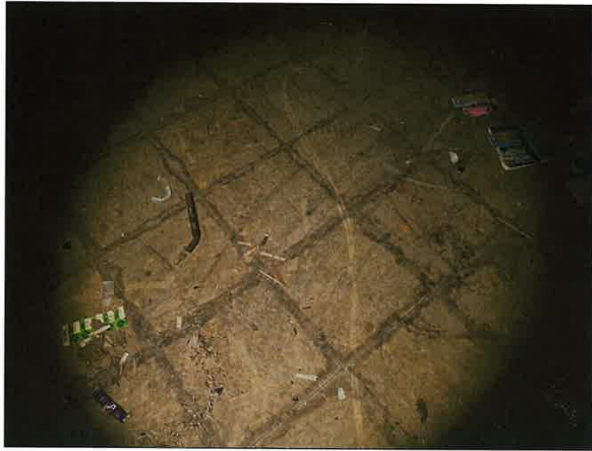
37 - Eastern Structure - ACM 12" x 12" Tan Floor Tile and ACM Black Mastic (FL1)
