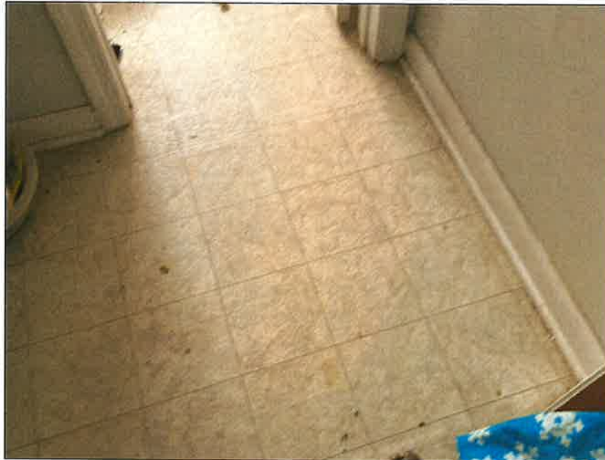
18 - Western Structure - Non-ACM Off-white Vinyl Sheet Flooring (FL6)
