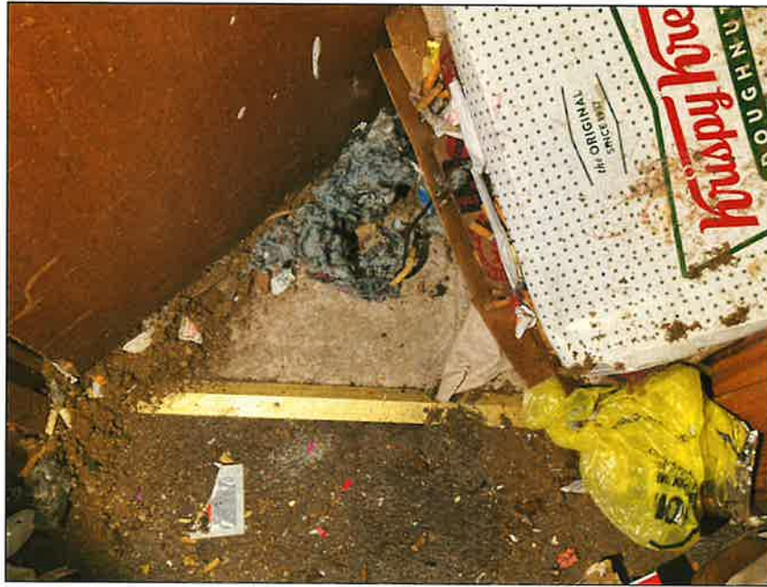
17 - Western structure - Non-ACM Pinkish-Grey Vinyl Sheet Flooring (FL5)
