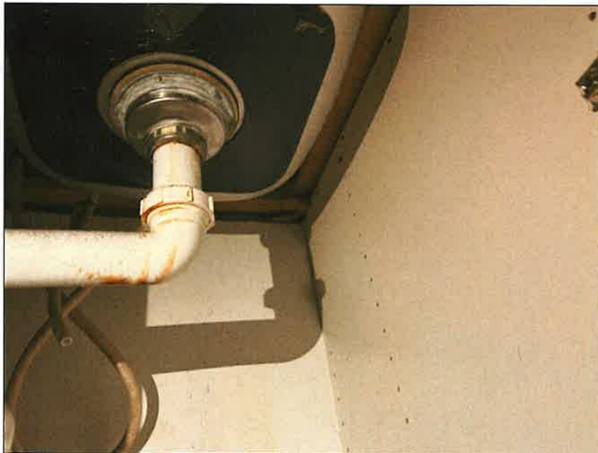
34 - Eastern Structure - Non-ACM Black Sink Underpad (SU1)
