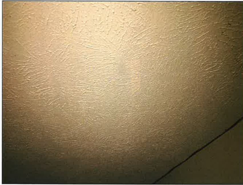
29 - Eastern Structure - Non-ACM White Ceiling Texture ("Stipple" Style) (CTX2)
