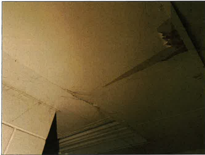
31 - Eastern Structure - Non-ACM 2' x 4' White Sanitary Ceiling Tile (CTL2)
