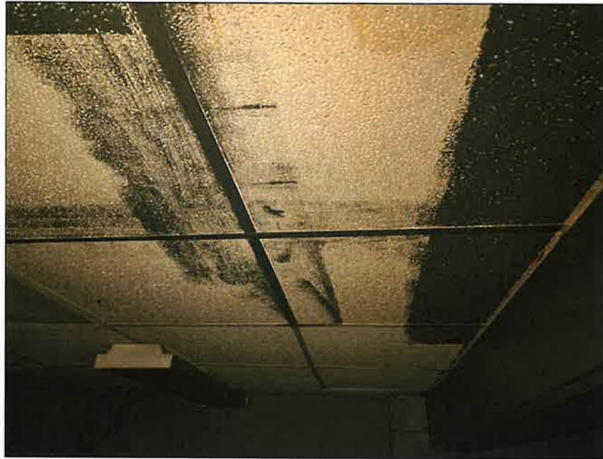
33 - Eastern Structure - Non-ACM 2' x 2' White/Grey Ceiling Tile (CTL4)
