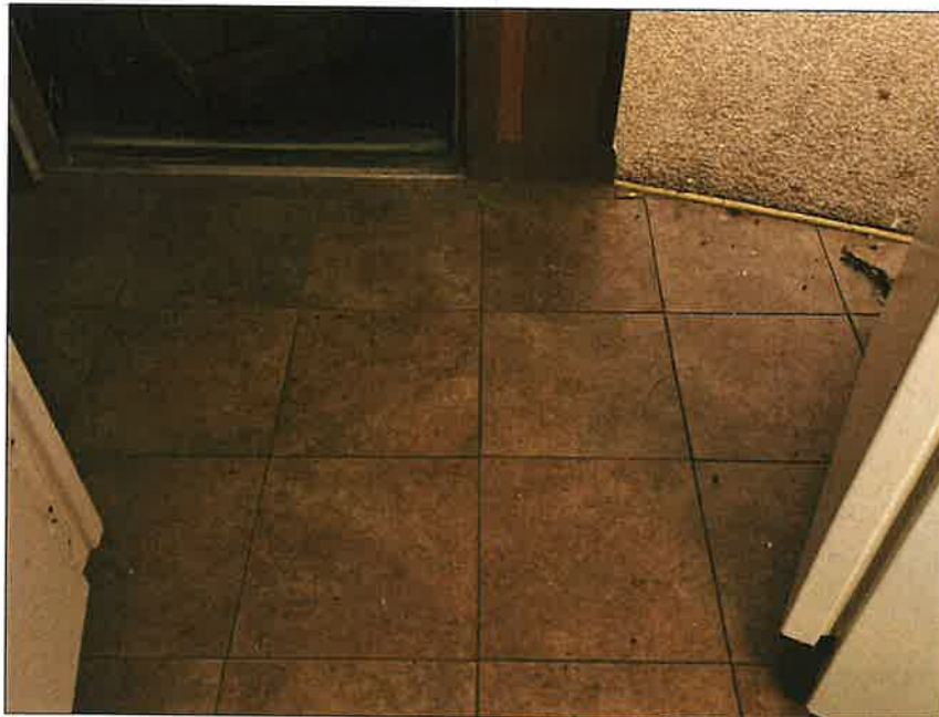
14 - Western Structure - Non-ACM Floor Tile with underlying ACM Vinyl Sheet Flooring (FL2)
