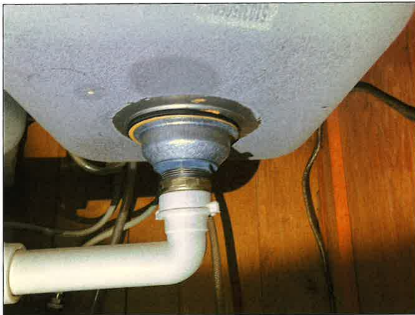
12 - Western Structure - Non-ACM Grey Sink Undercoating (SU1)
