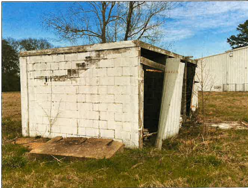
20 - Center Structure - Non-ACM White/Grey CMU Coat (CO1)
