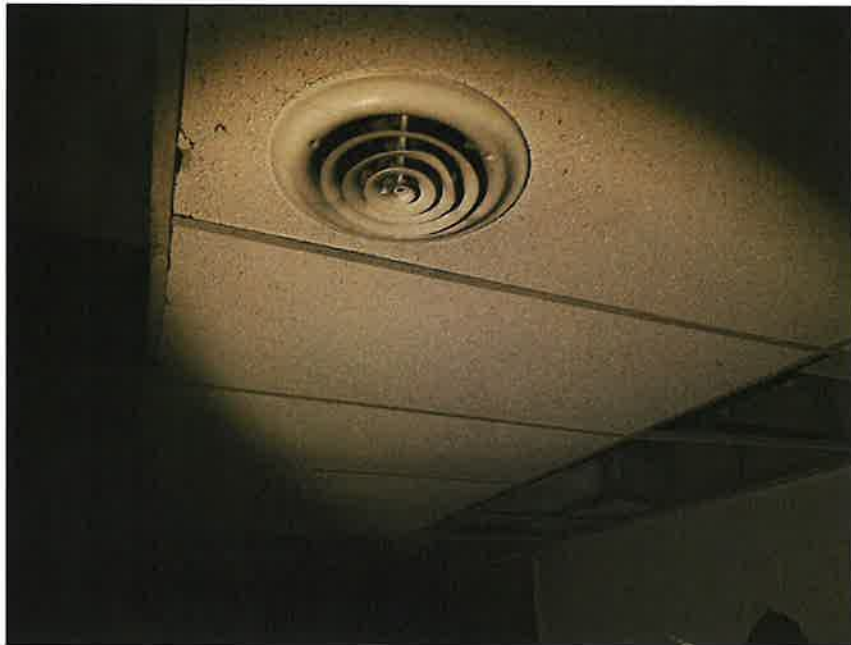
30 - Eastern Structure - Non-ACM 2' x 4' White Ceiling Tile (Pinholes and Fissures) (CTL1)
