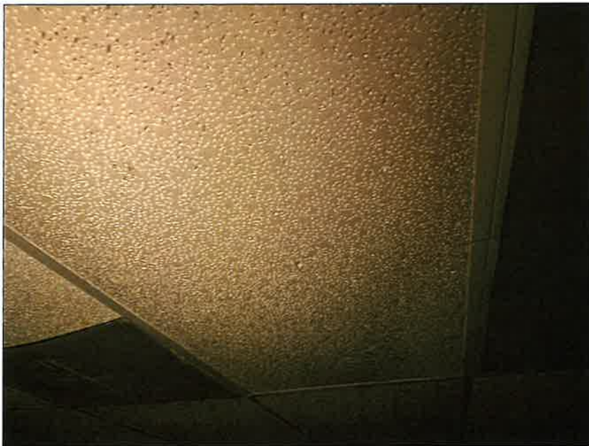
32 - Eastern Structure - Non-ACM 2' x 4' White Ceiling Tile (Small and Large Holes) (CTL3)
