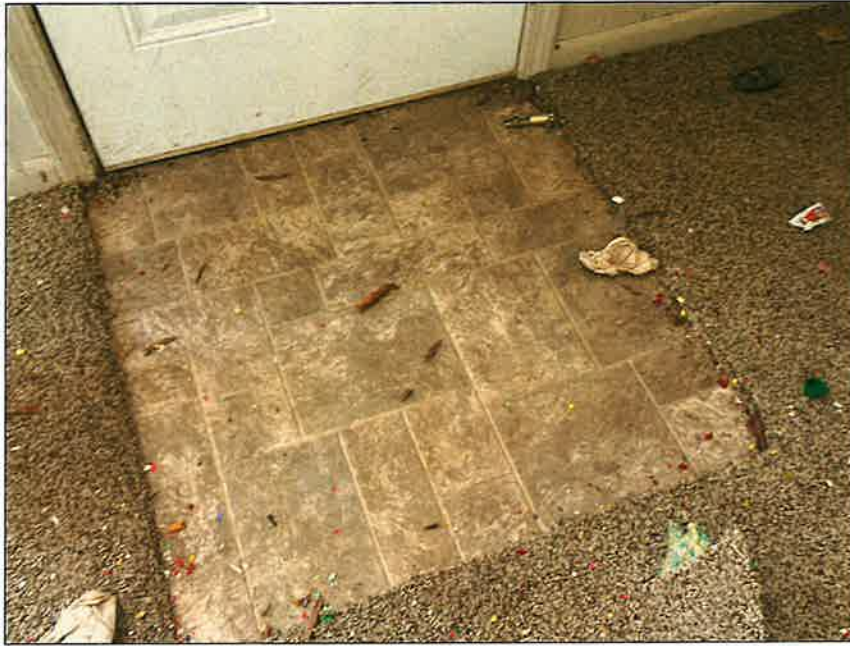
15 - Western structure - Non-ACM Vinyl Sheet Flooring atop ACM Vinyl Sheet Flooring (FL3)
