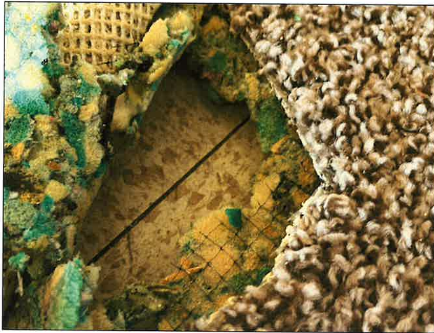
13 - Western Structure - ACM 12" x 12" Tan Floor Tile and Mastic (FL1)
