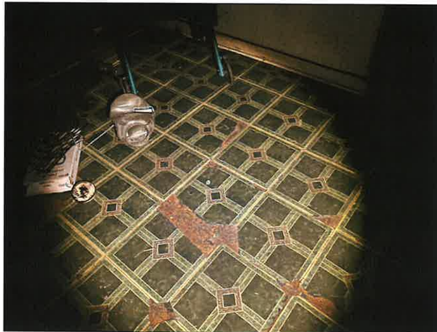
38 - Eastern Structure - Non-ACM Vinyl Flooring, located in Floor 1 Southern Area Bathrooms (however, ACM black mastic was observed underneath the materials)
