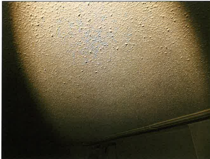
28 - Eastern Structure - ACM White Ceiling Texture ("Popcorn" Style) (CTX1)
