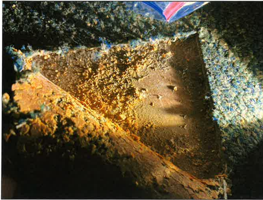
39 - Eastern Structure - Non-ACM Yellow Carpet Mastic (CM1)
